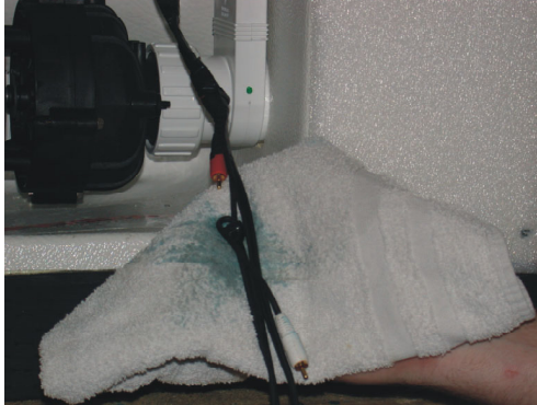
Figure 16. Applying Lubricant to Cables
